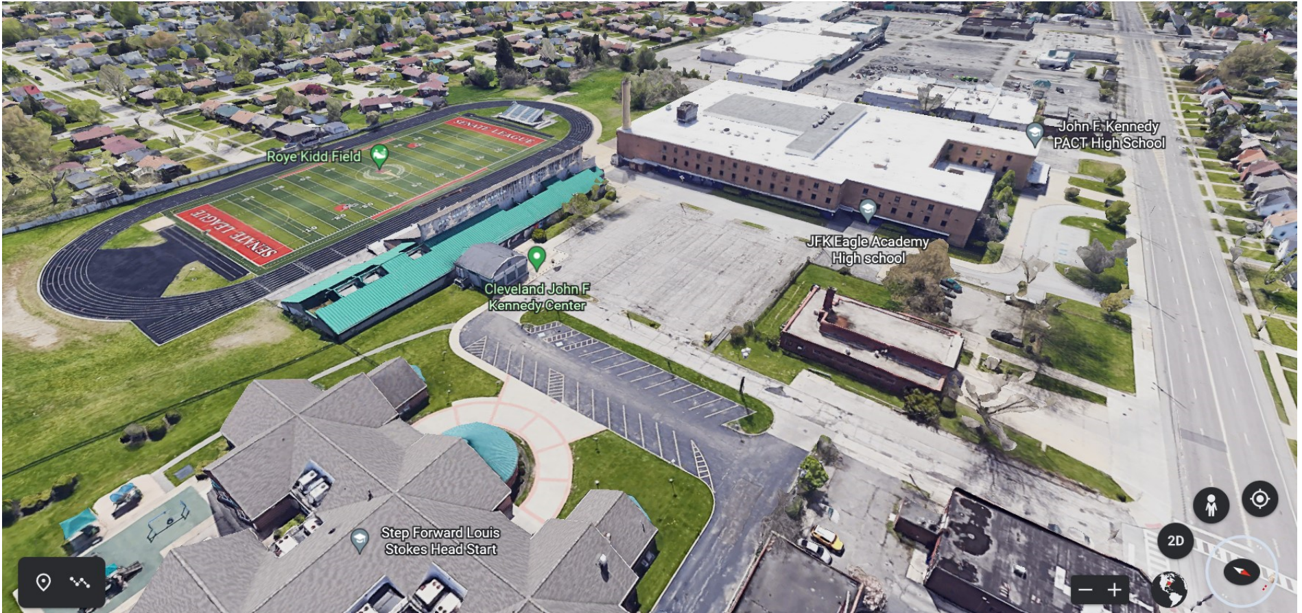
Site Aerial View
