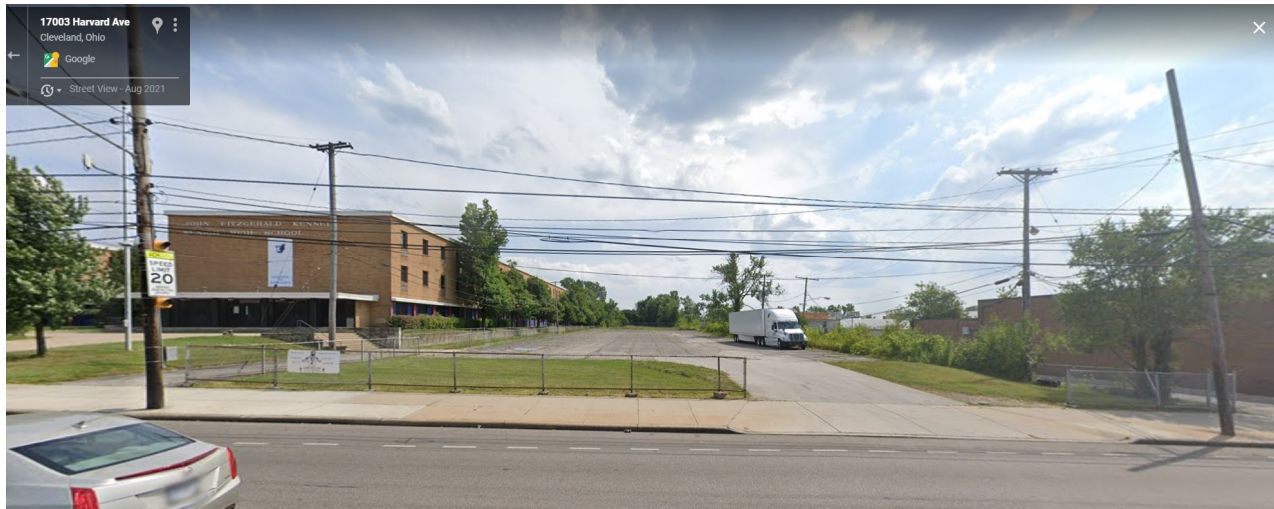
Existing Exterior Views – JFK HS
