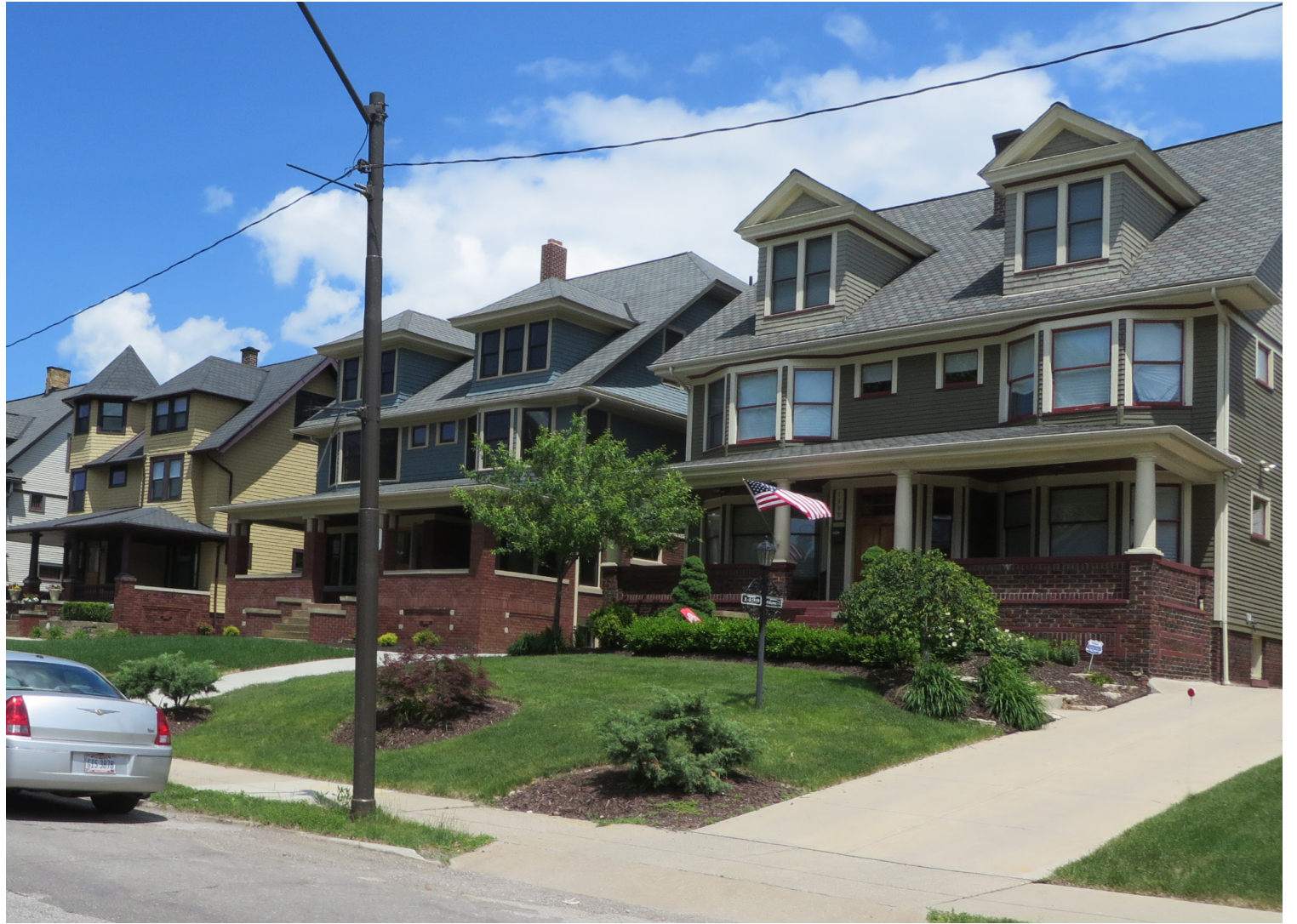
The Heritage Lane section of E 105th Street extends economic activity north of University Circle.
