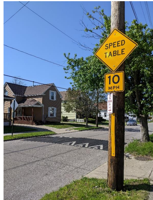
Figure 1 Speed Table Installation on W. 56th Street
